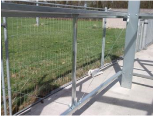
Anti sag system as required by BS5950
