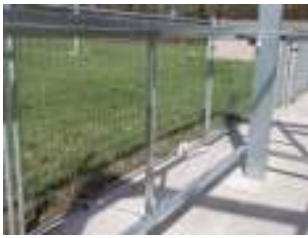
Anti sag system as required by BS5950
