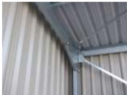
Anti condensation lining on all single skin roof panels
